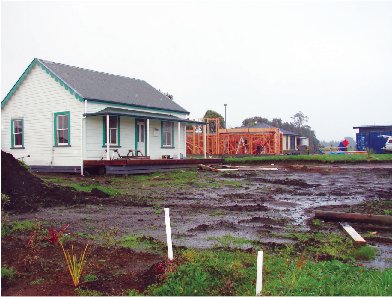
A contrast - one house relocated while another is under construction.
